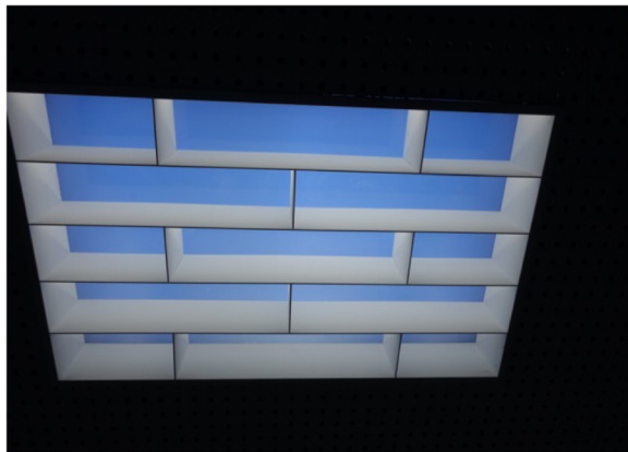
Fig. 2 Artificial skylight seen from below
